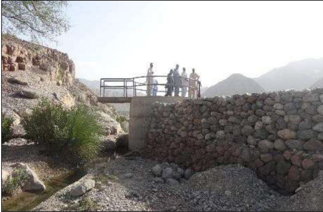
Figure 3: Existing intake structure
