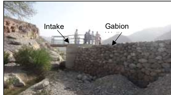
Figure 8- Existing intake structure and flood protection gabion wall
