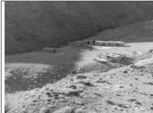
View of the rooms (animal sheds) to be inundated at Killi Landi
