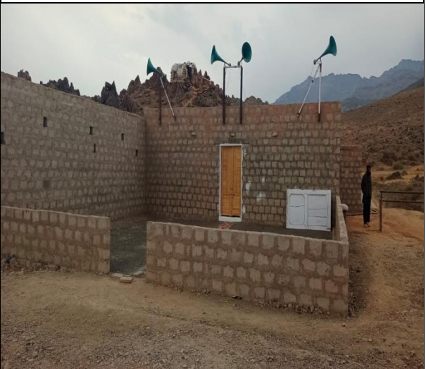
Mosque under construction for prayers.
