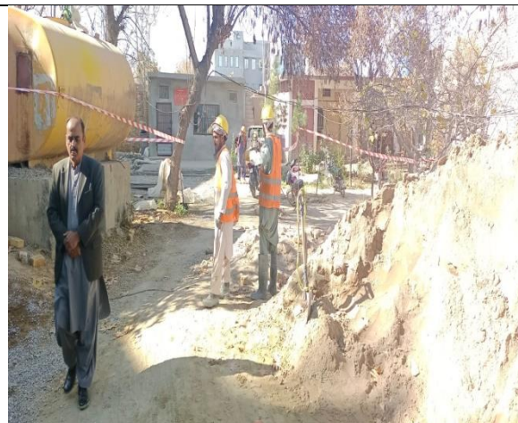
Workers using PPE's on site
