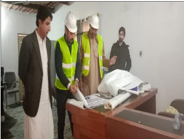
Safety signboards panaflex arrived during field visit at Siri Toi Dam Camp.
