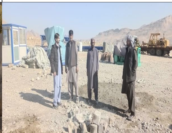
Installation or erection of batching plant on selected site
