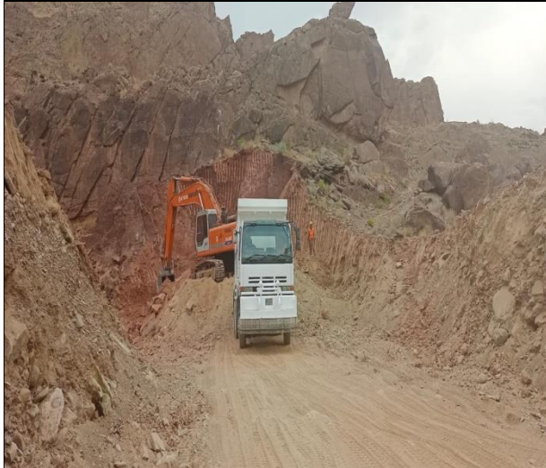
Excavation of Dyke (Earth work).
