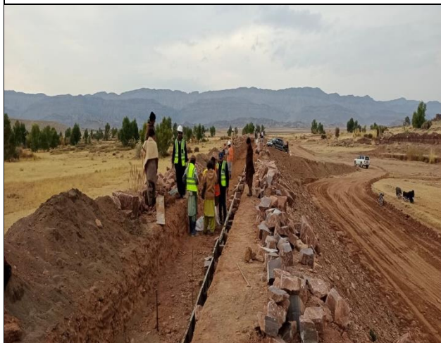
Workers using PPE's at site.
