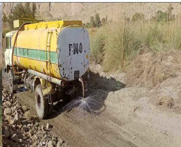
Onsite water sprinkling on bund 3A.
