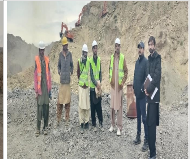
Joint visit of SC Environmental Specialist along with Contractor Environmental Specialist.
