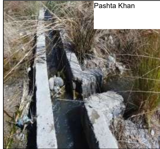
Figure 5-2: Existing lined Channel
