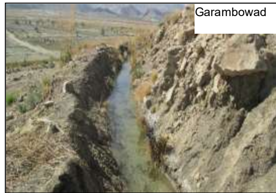
Figure 5-4: Earthen channel for Garambowed command area
