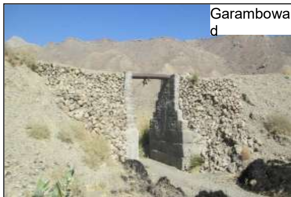
Figure 5-5: Pipe aqueduct on Garambowad channel
