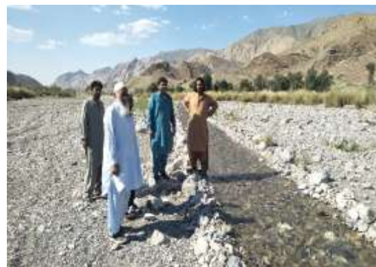
Figure 5-6: Upstream guide channel for diversion bund of Garabowed
