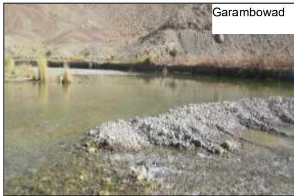
Figure 5-3: Earthen diversion bund for Garabowed
