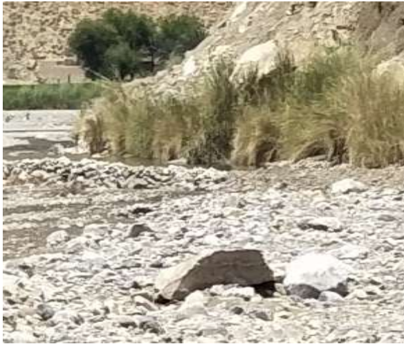
Figure 5-1: Existing bund for diversion of flow
