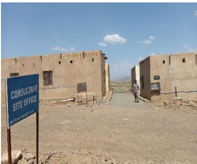
Figure 6: Consultant Site Office
