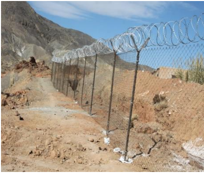
Figure 32: Fencing around the site area
