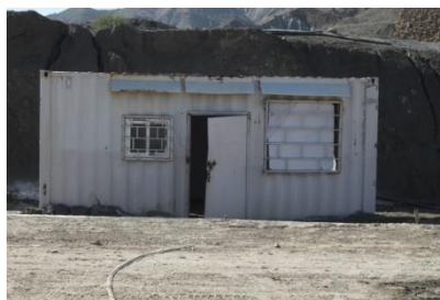
Figure 5: Consultant Camp Office
