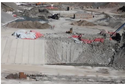
Figure 2: Stock Piles at Site
