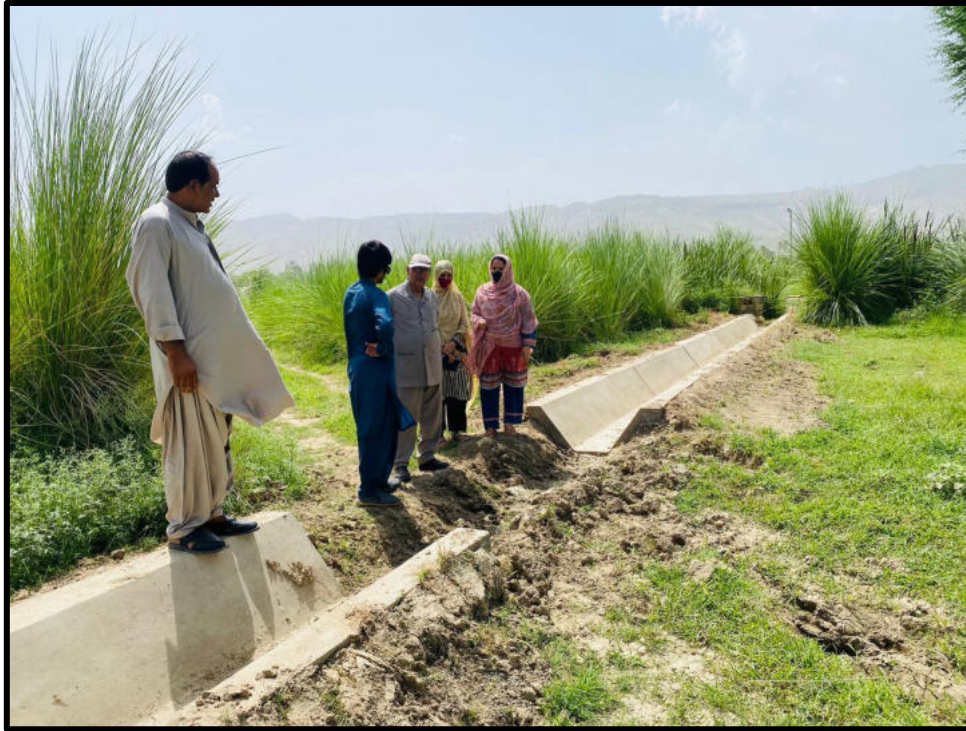
Figure 4: Visit to the Watercourse under construction Scheme at MRB Karakh District
