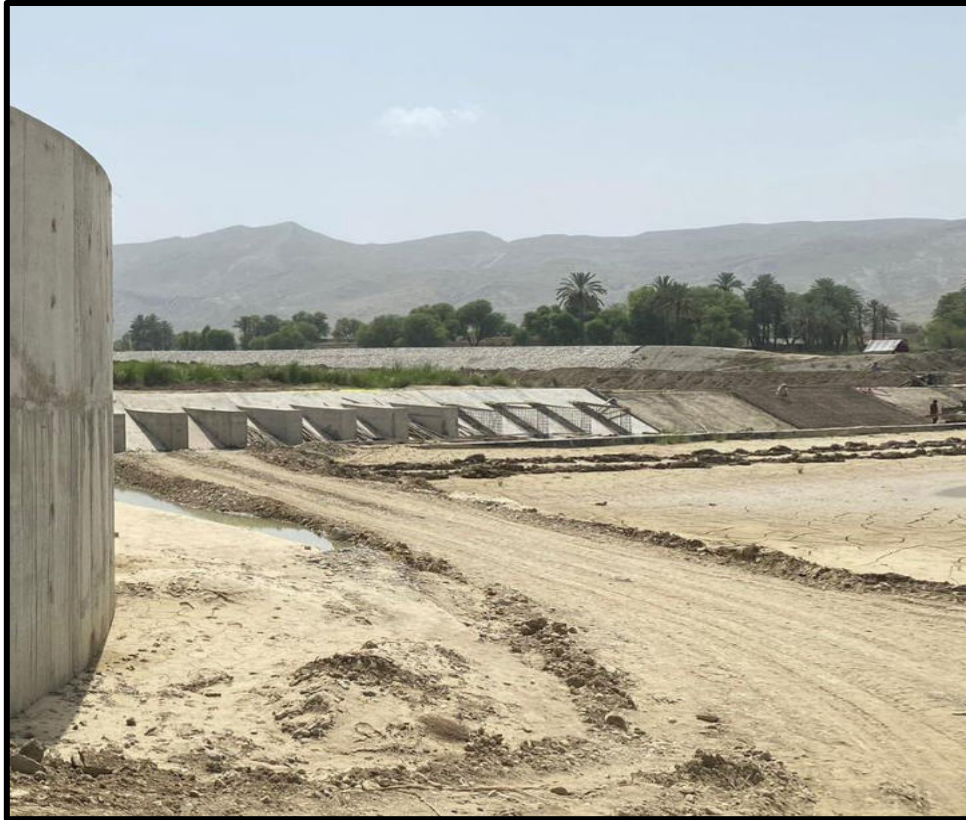
Figure 8: Under construction Weir near Village Wandhri District Karakh
