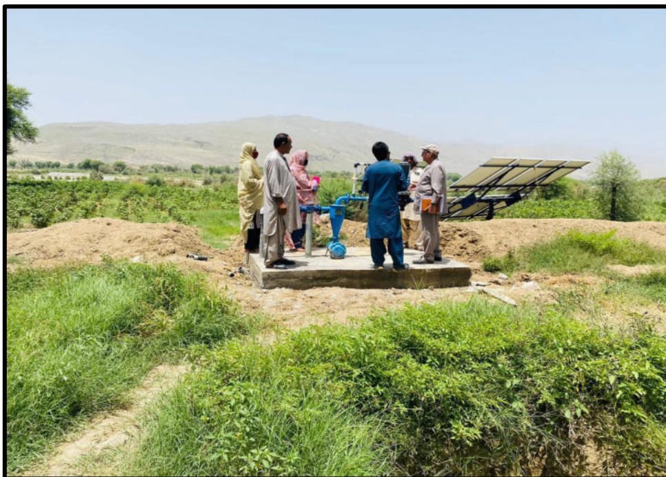
Figure 3: Installed Solar Power Drip Irrigation System at Wandhari Karakh District
