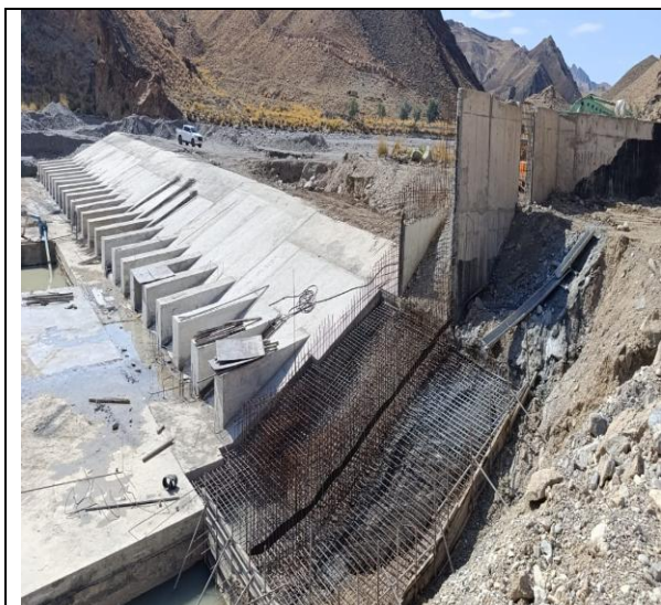
Construction on Pashta Khan Grambowad Subproject NCB-04, MRB
