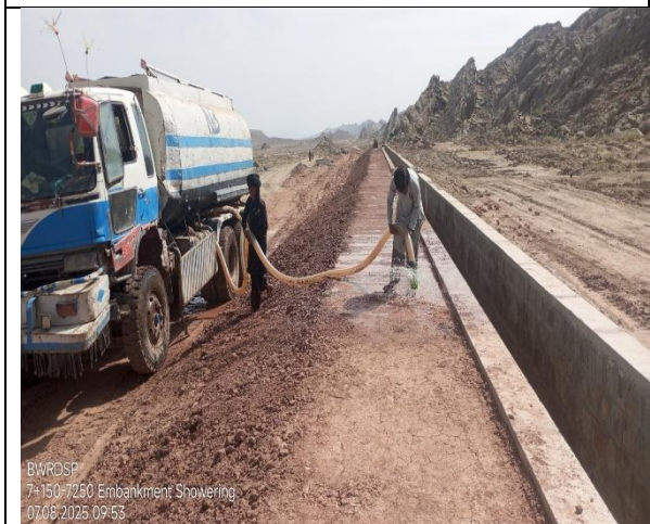
Construction of RBC under ICB-01, ZRB
