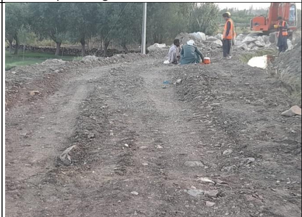
Flagmen present on approach road where construction activity is in progress
