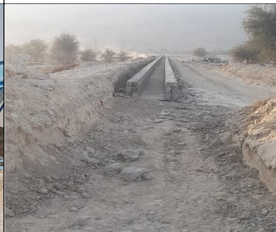
Construction of Chutta Main sump No.1
