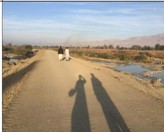
Movement of vehicles was noticed during site visit on Bund No.1. Water sprinkling is greatly required. Contractor team was advised to provide water tanker to reduce dust pollution.
