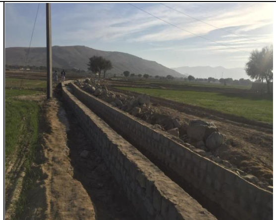
Stone Masonry work in progress on irrigation channel
