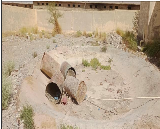
Empty drums present within the vicinity of camp site, contractor team was advised to properly reuse these drums in any positive activity.
