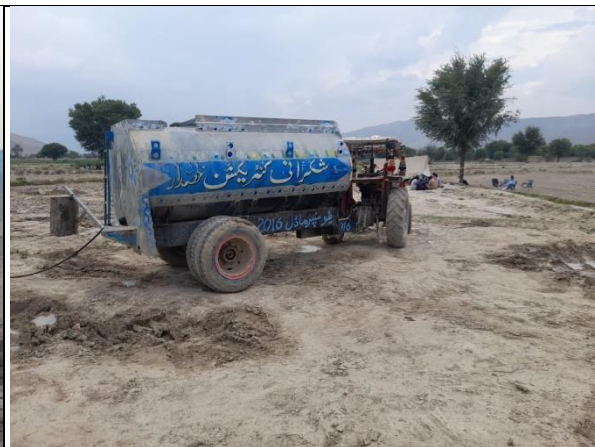
Water sprinkling to reduce dust emission
