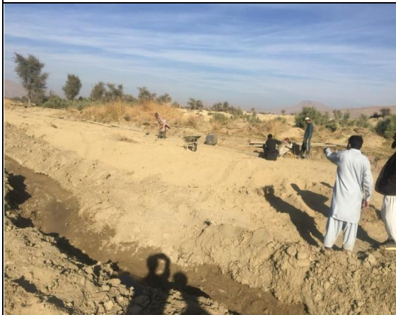
Environmental Specialist addressing contractor to provide proper PPE's to site workers
