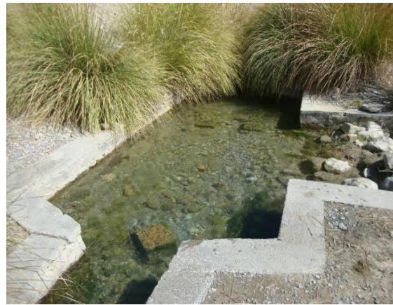
Existing Hitachi Channel d/s of Syphon
