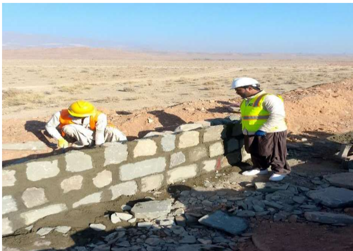
Figure 3-2: Works Progress in Pictures
