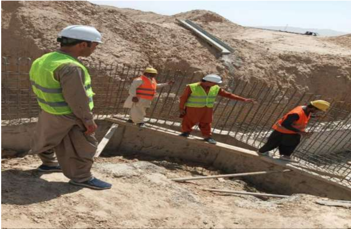
Figure 4-2: Construction of Pashta Kha D/S Weir Panel No .5 in Progress
