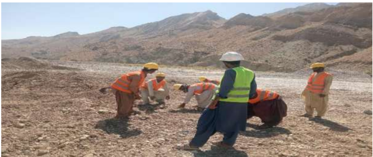
Figure 5-2: On going Construction activities at NCB-07
