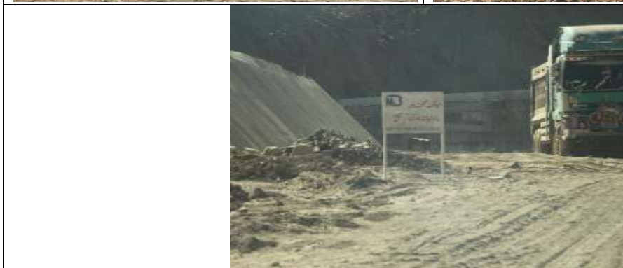
Safety Signboard at Site
