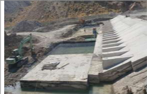
No Caution Tapes are installed around the excavated areas
