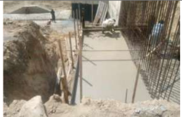
No Caution Tapes are installed around the excavated areas
