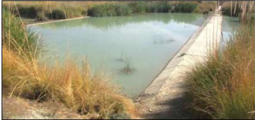
Figure 4: View of Khadri Weir
