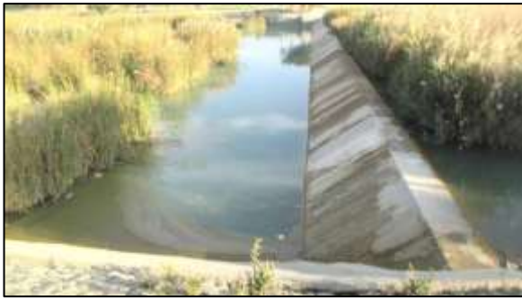
Figure 6: View of Acherwand Weir
