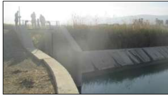
Figure 7: View of Channel Off-take point of Acherwand Weir
