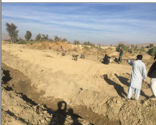
Environmental Specialist addressing contractor to provide proper PPE's to site workers
