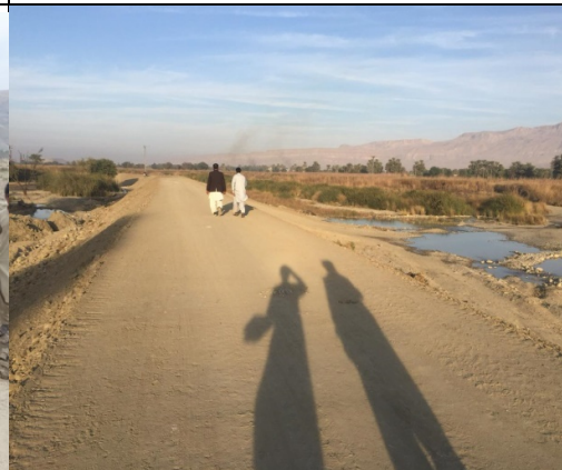
Movement of vehicles was noticed during site visit on Bund No.1. Water sprinkling is greatly required. Contractor team was advised to provide water tanker to reduce dust pollution.
