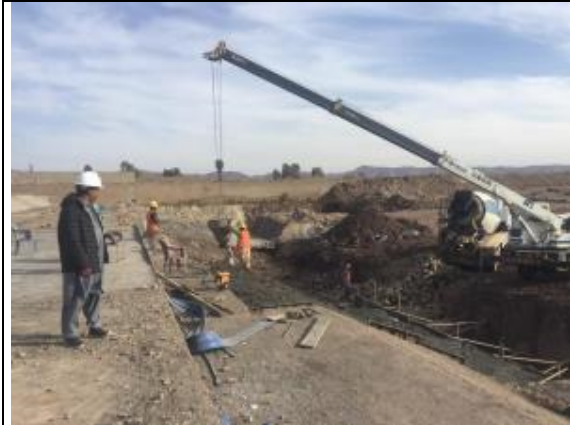
Workers using PPE's during construction activities
