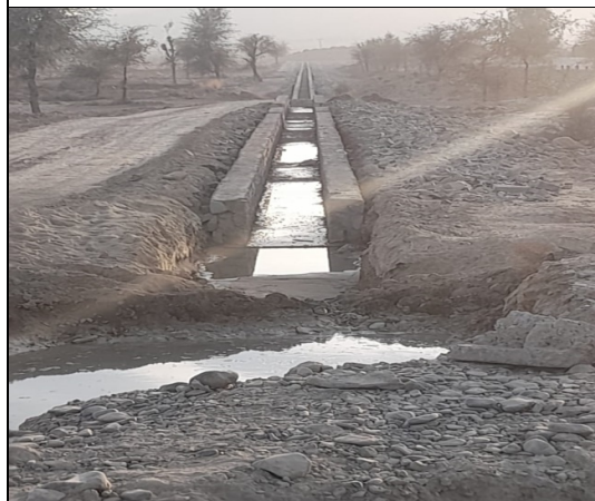
Construction of Chutta Left sump No.1
