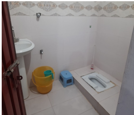
Contractor officials washrooms in hygienic condition
