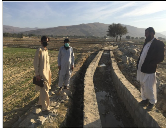
Stone Masonry work in progress Wandri left Irrigation Scheme
