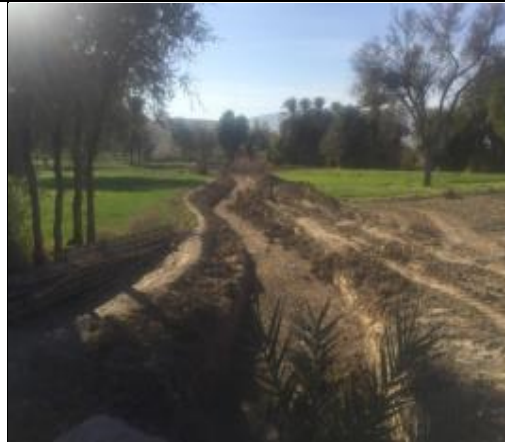
Excavation/Earth work in progress on Acherwand Irrigation scheme
