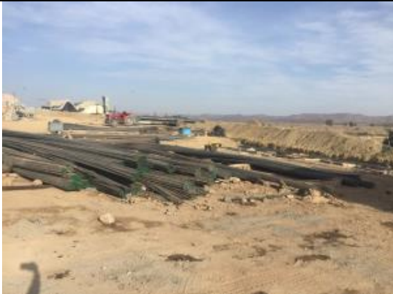
Steel should be covered with polythene sheet to avoid rusting
