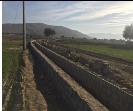
Stone Masonry work in progress Wandri Right Irrigation Scheme
