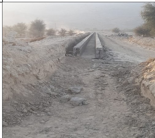
Construction of Chutta Main sump No.1
