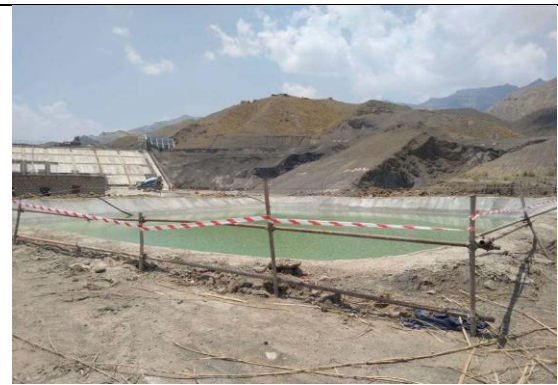
Site Safety Barricade
