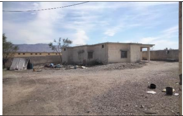
Poor Hygiene condition at Camp
