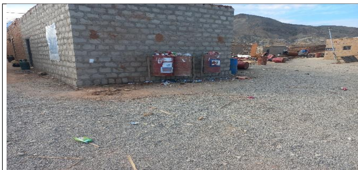
Solid Waste overflowing bins in Siri Toi Dam Camp site
