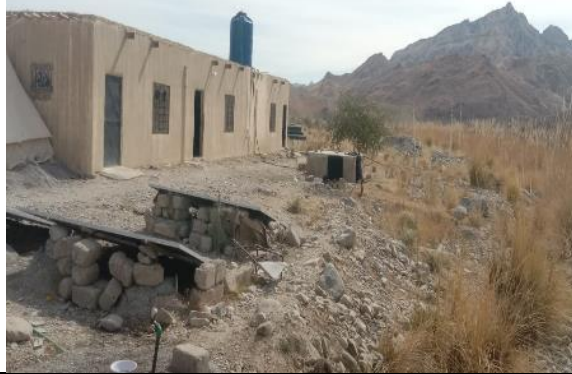
Poor utilities setup at camp
