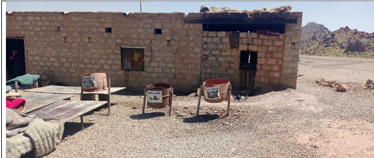
Presence of signboards for adequate disposal of waste at Camp site
