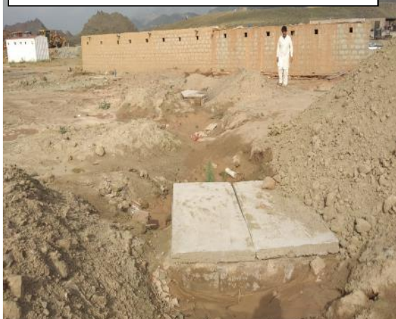
Septic Tanks constructed in camp area
