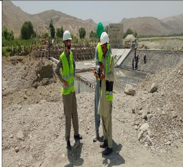
Ambient air test at Karkh construction site
