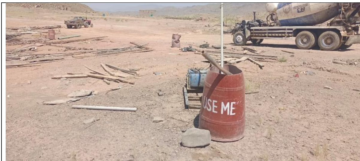
Waste bin provided on construction site
