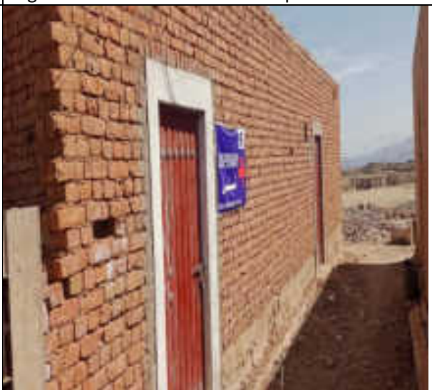
Dispensary in Contractor camp
