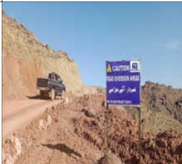
Precautionary signboard at diversion point
