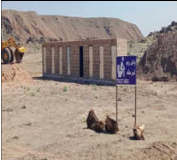
Ensuring presence of signboards mentioned in CAP
