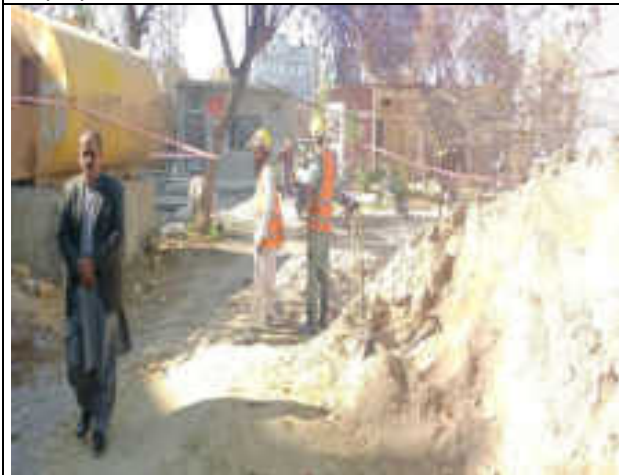
Workers using PPE's on site
