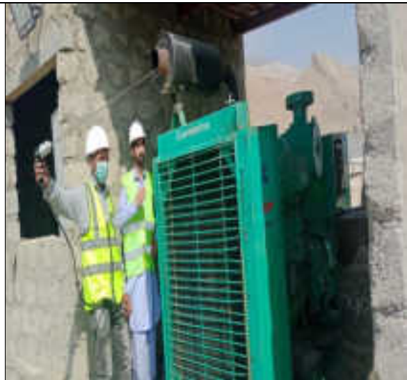
Gaseous emission monitoring on construction site
