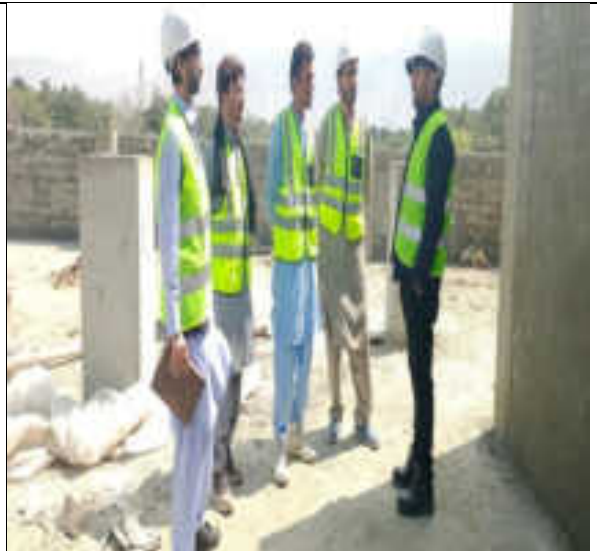
Discussion on PPE's with Contractor Environmental Specialist
