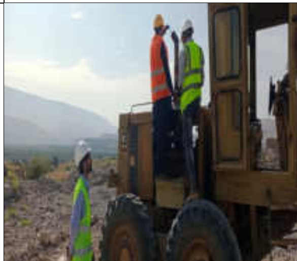
Gaseous emission monitoring on construction site
