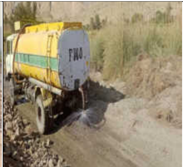
Onsite water sprinkling in process
