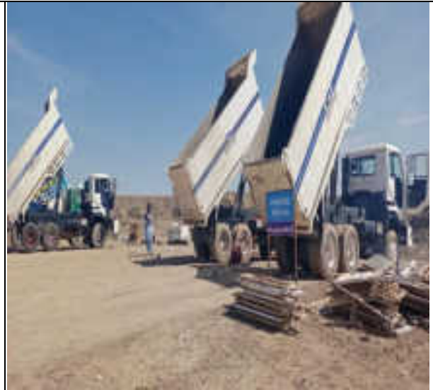
Ensuring presence of signboards mentioned in CAP of Siri Toi Dam
