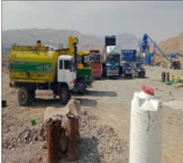
Vehicles parking area
