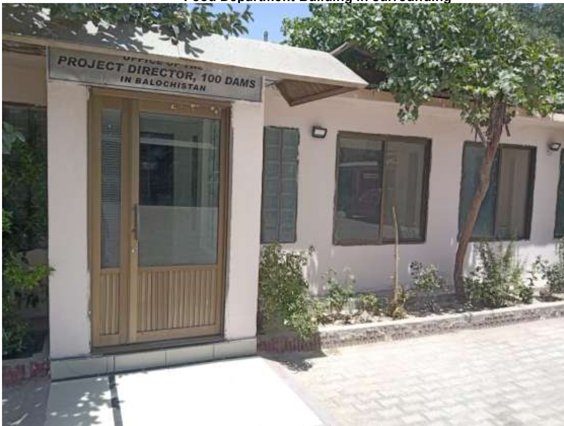
Project Director, 100 Dams project office adjacent to Proposed project site
