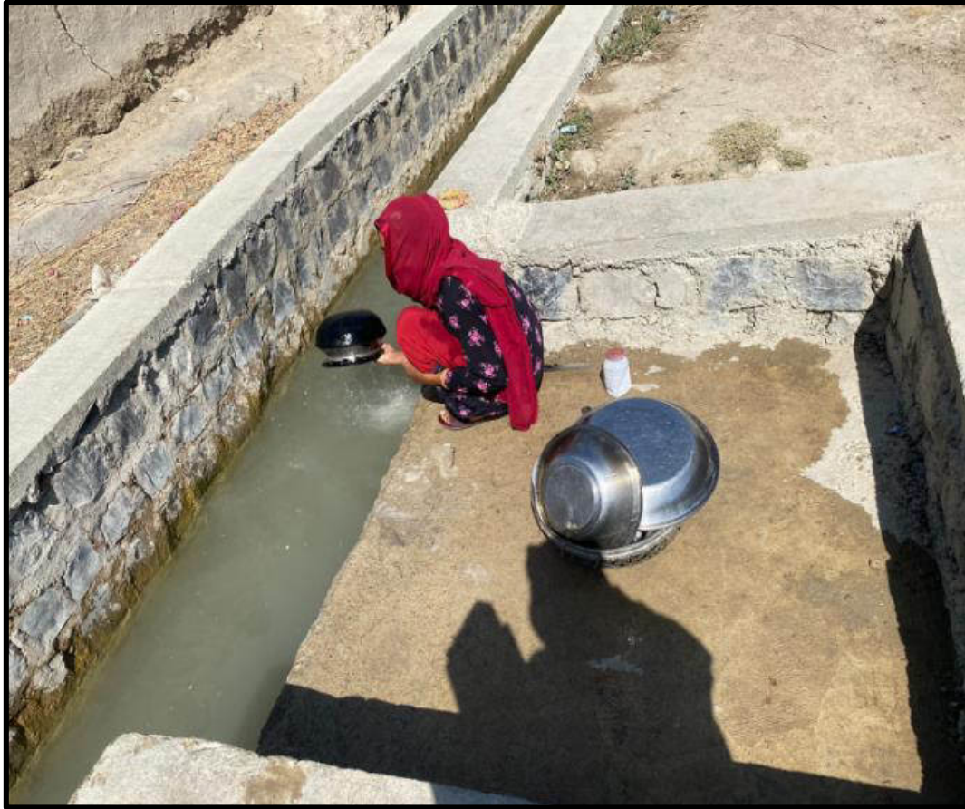
Figure 5-5: Washing Pads Structures for Women Facilitation
