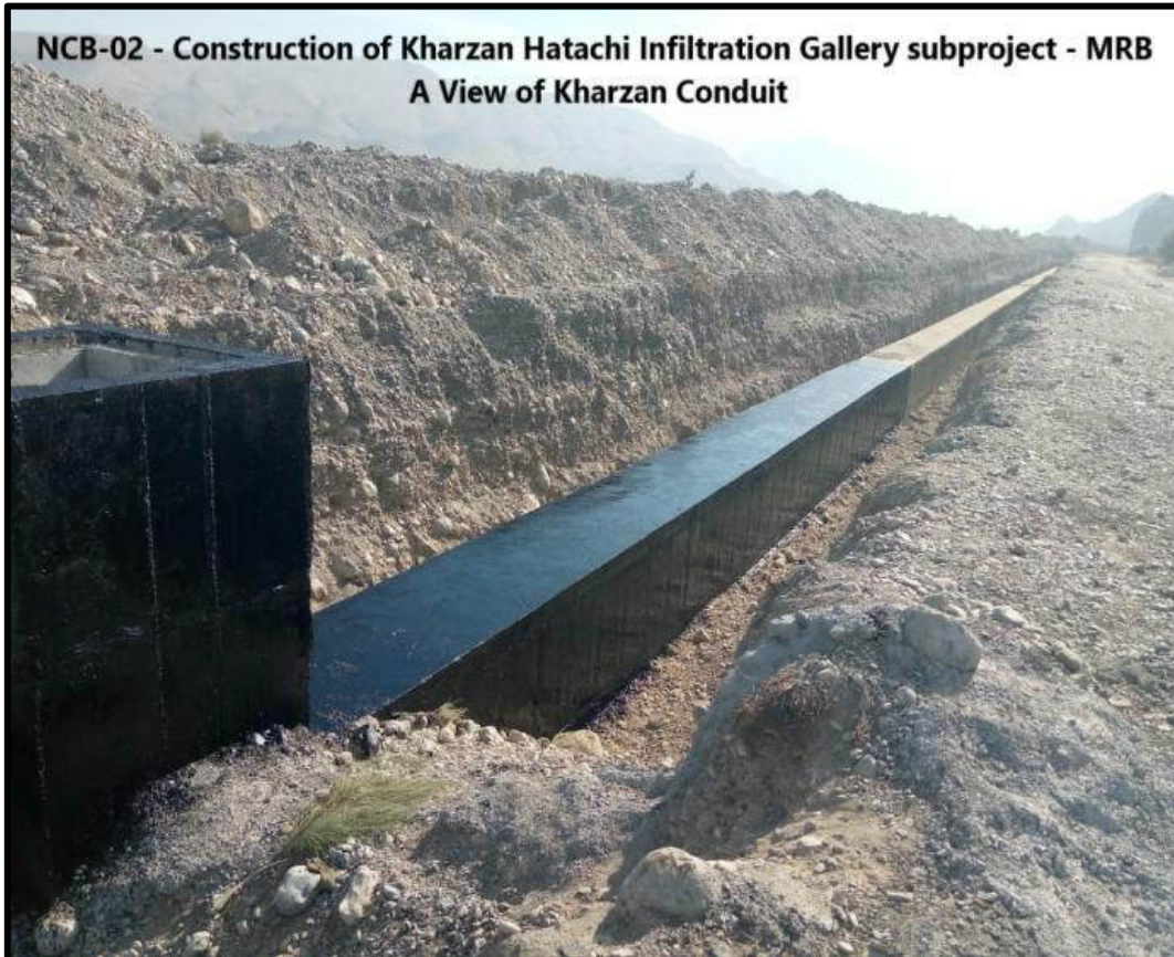
Figure 5-3: Kharzan Hatachi Infiltration Gallery (NCB- 02) Sub-Project Work In Progress
