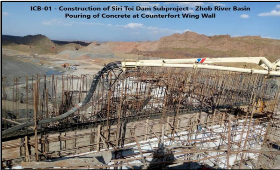
Figure 5-1: Construction Activities of Spillway of Siri Toi Dam
