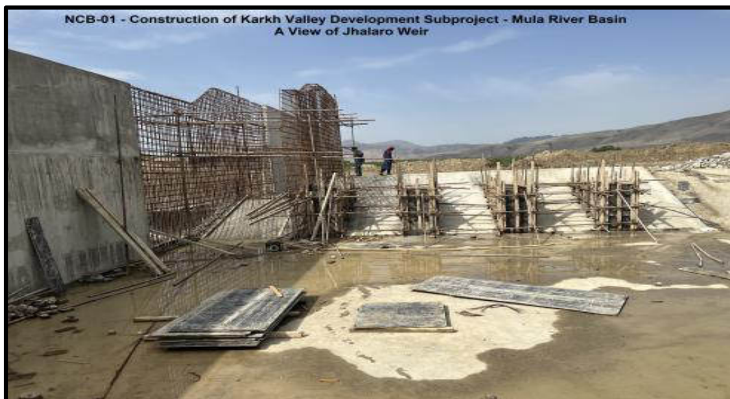
Figure 5-2: Karkh Valley FIS (NCB- 01) Sub-Project Work in Progress
