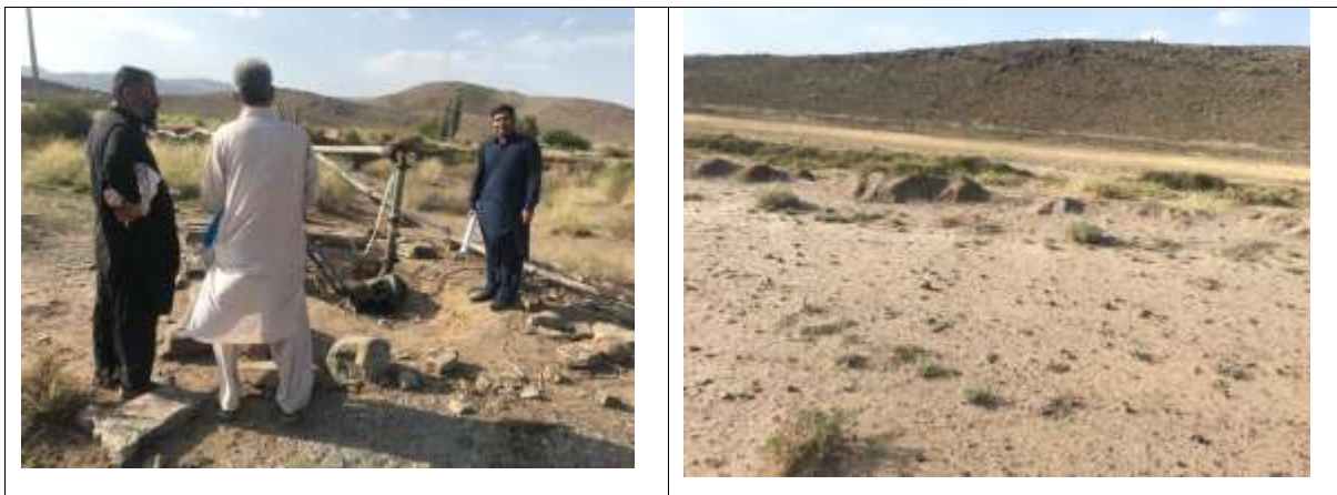
Figure 6: Irrigation Trough Diesel Engine (Tube Well) and Killi Sardar Akhtar Zai Subproject Command Area
